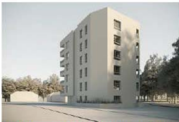
Figure 74: View 01 - Approach from west of Fairchildes Avenue
